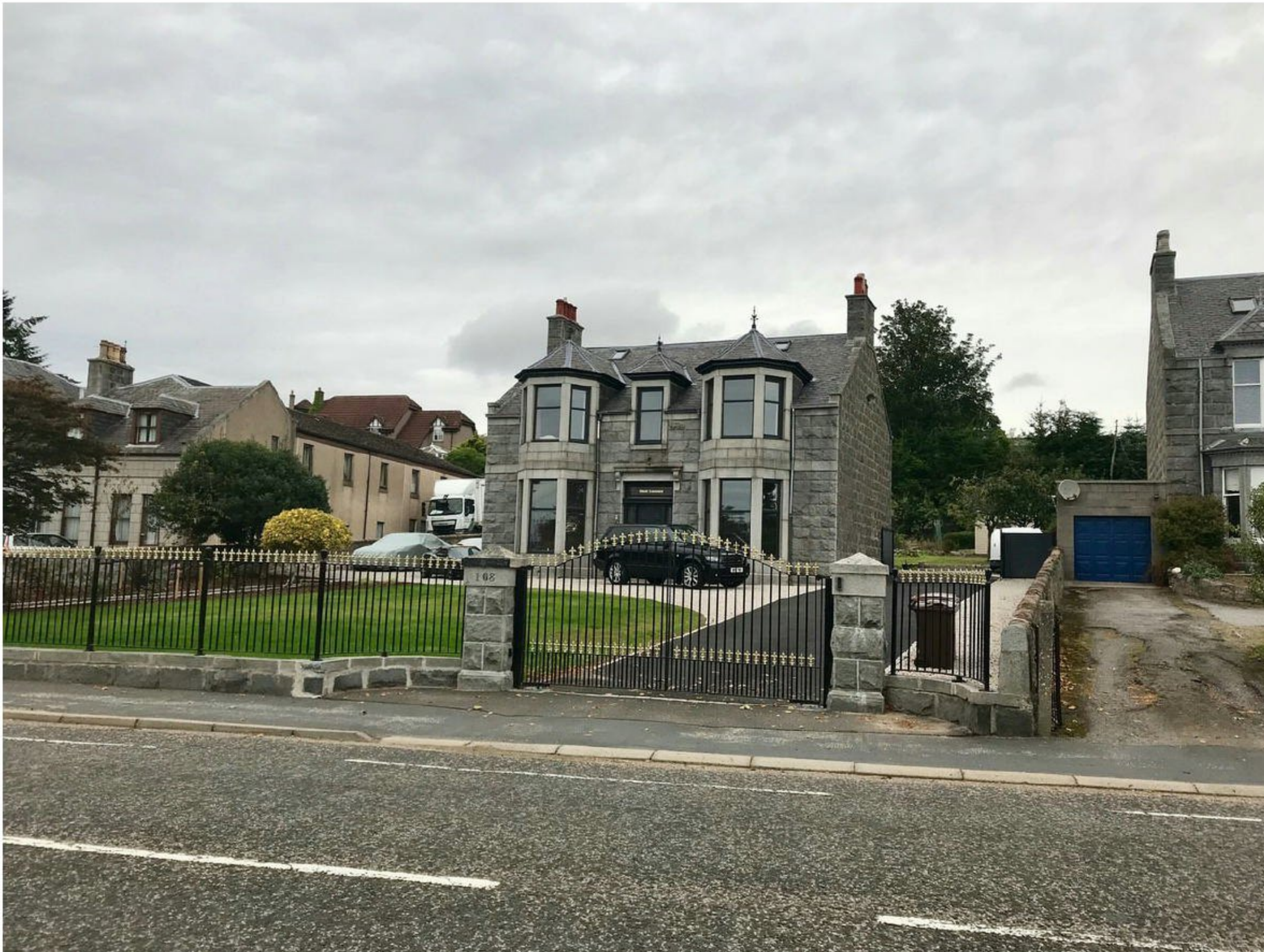
Figure 2 - 108 North Deeside Road with 10m wide gable.
